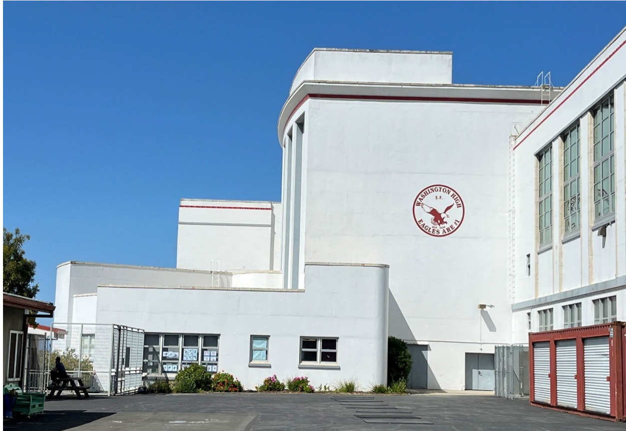
Photo 11. East façades of Music Wing Addition (left) and Auditorium (right), camera facing west.
