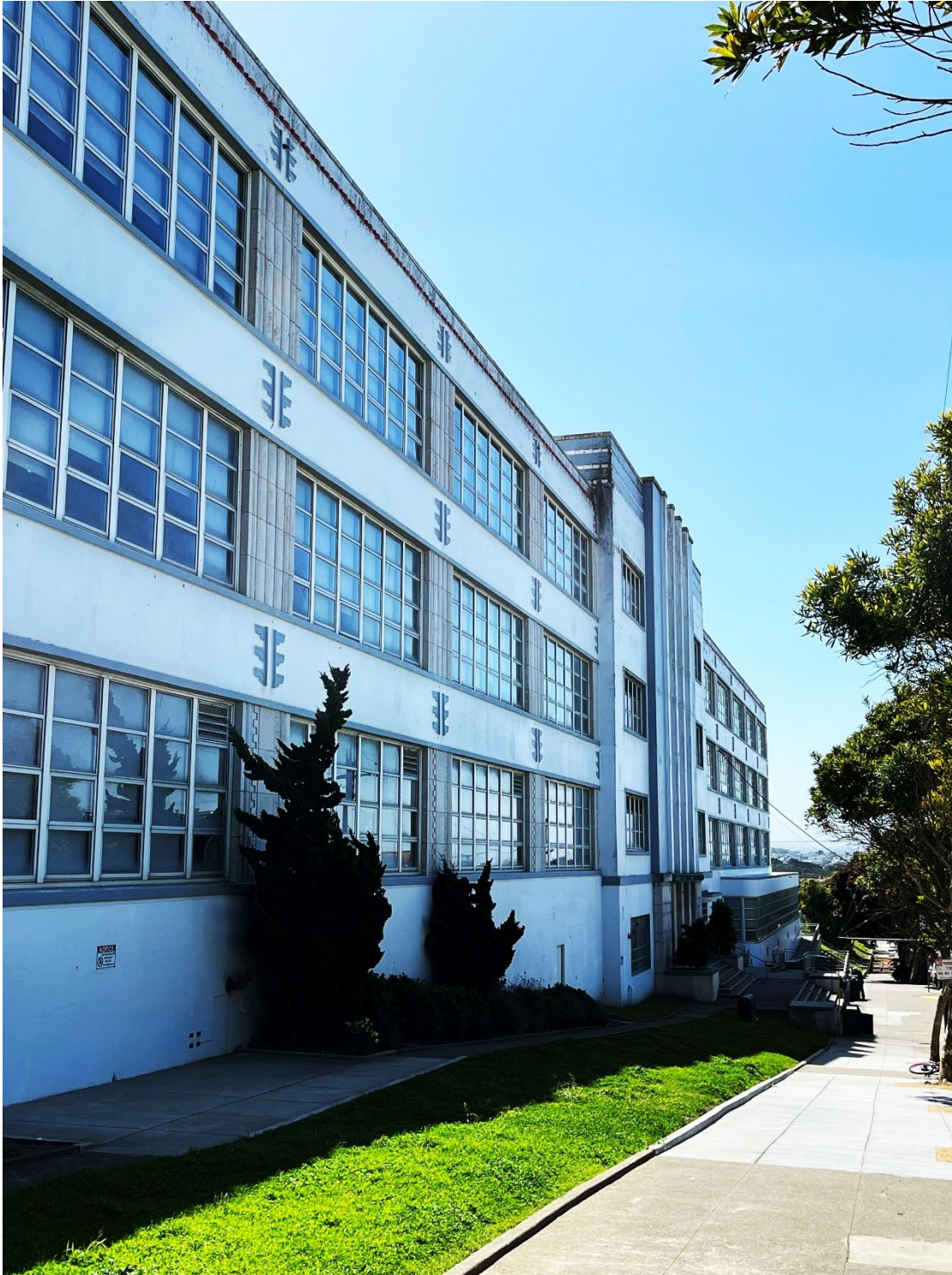
Photo 1. Overall perspective of west (primary) façade of Academic Building, camera facing south.
