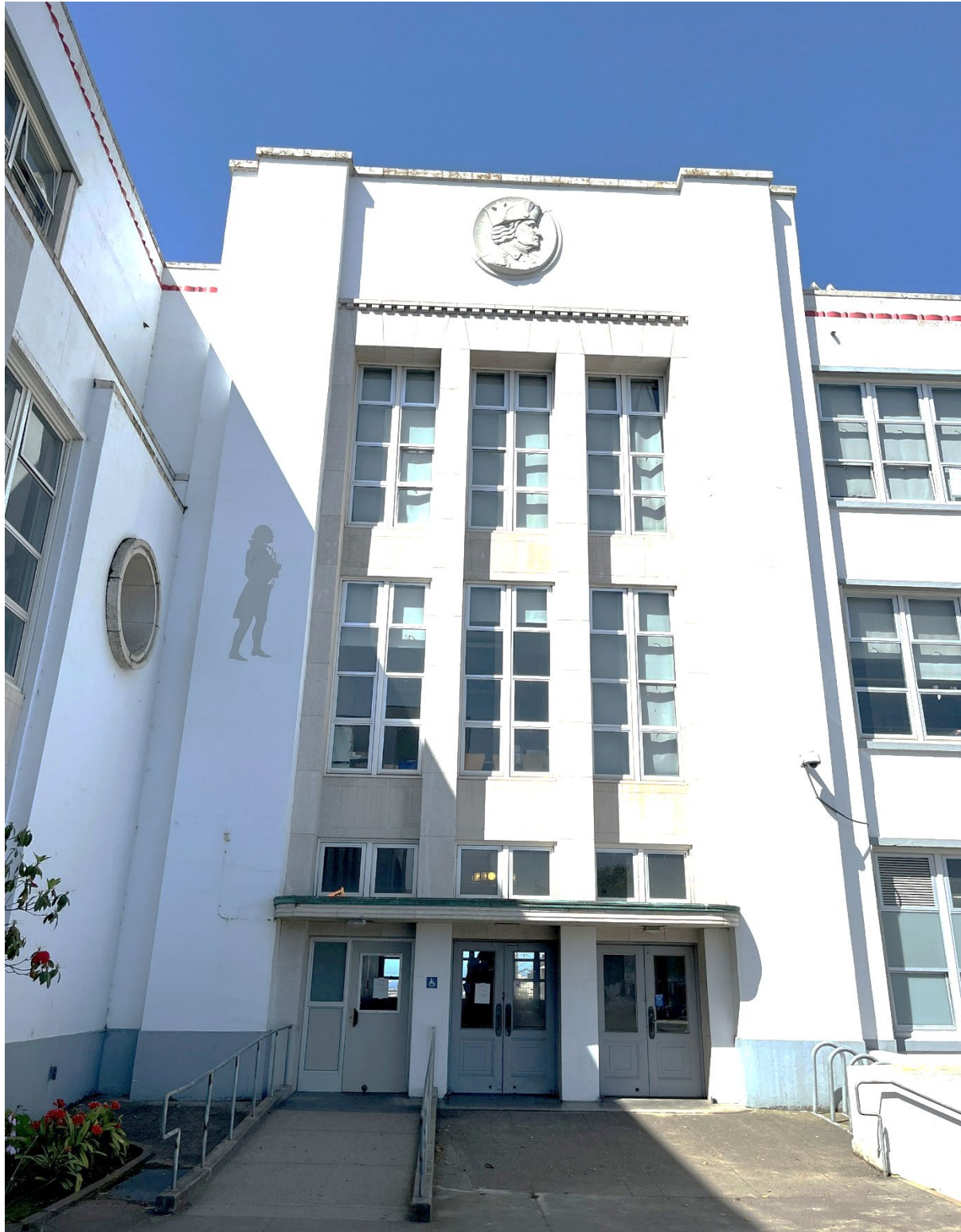
Photo 7. Detail of rear entrance on east façade of Academic Building, camera facing west.
