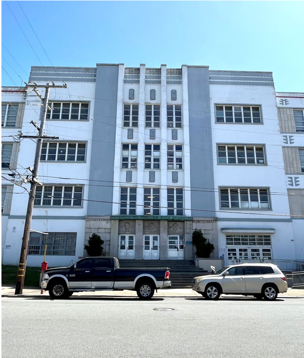
Photo 2. Detail of west (primary) façade of Academic Building, camera facing east.
