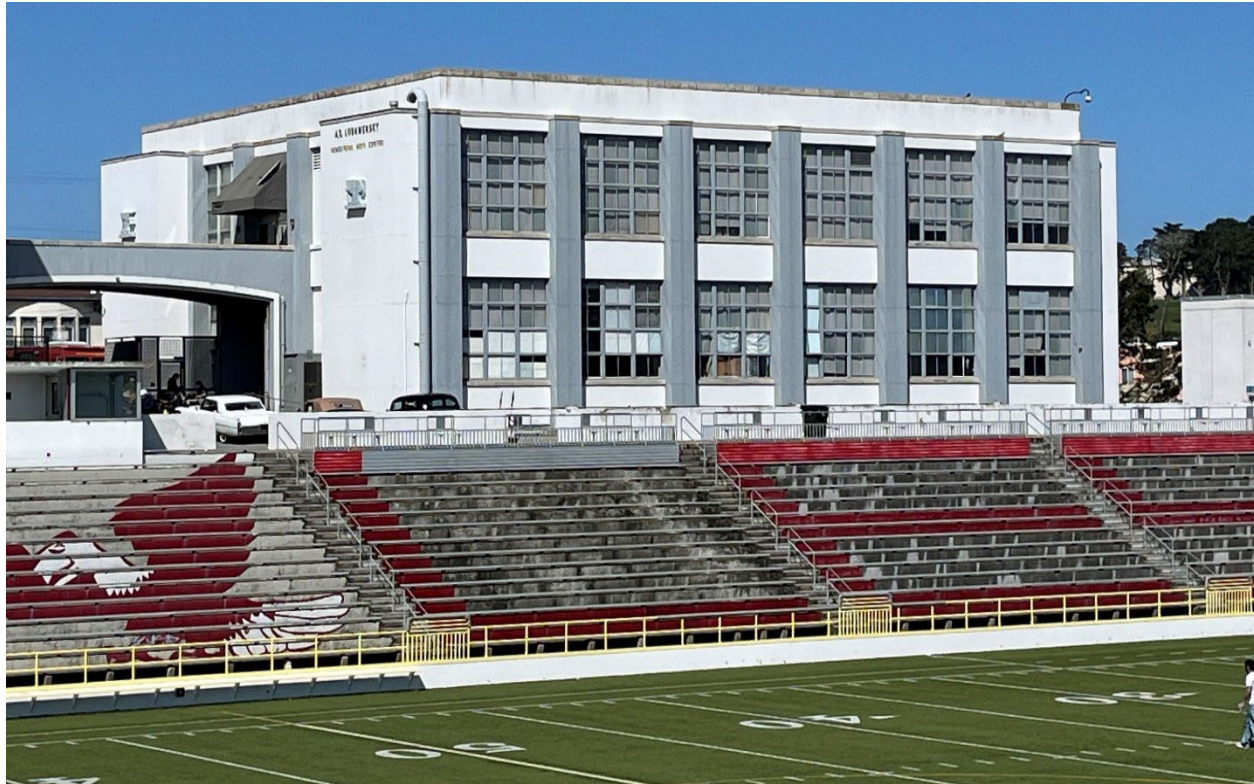
Photo 13. South and east façades of Shop Building, camera facing northwest.
