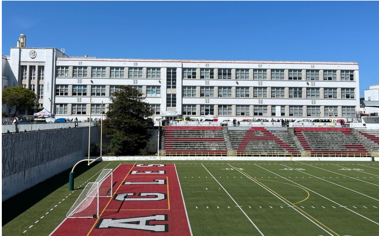
Photo 6. East façade of Academic Building, camera facing west.
