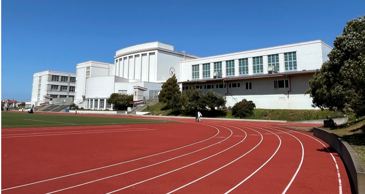
Photo 18. Track, camera facing northwest.
