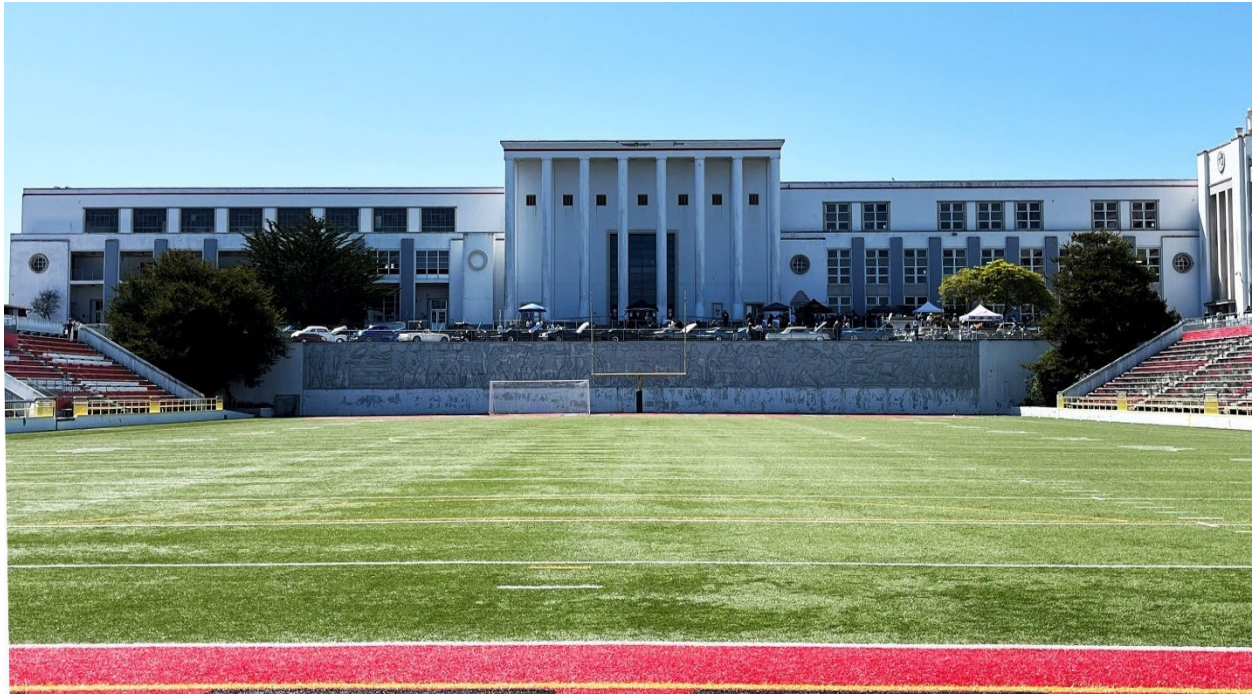
Photo 5. North façade of Gymnasium (left), Auditorium (center), and Academic Building (right), camera facing south.
