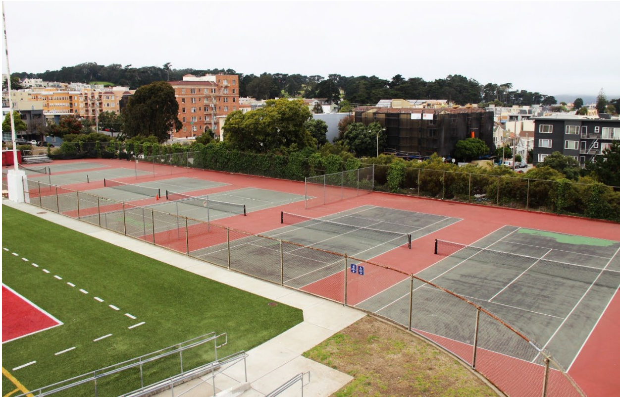
Photo 17. Tennis courts, camera facing northwest.
