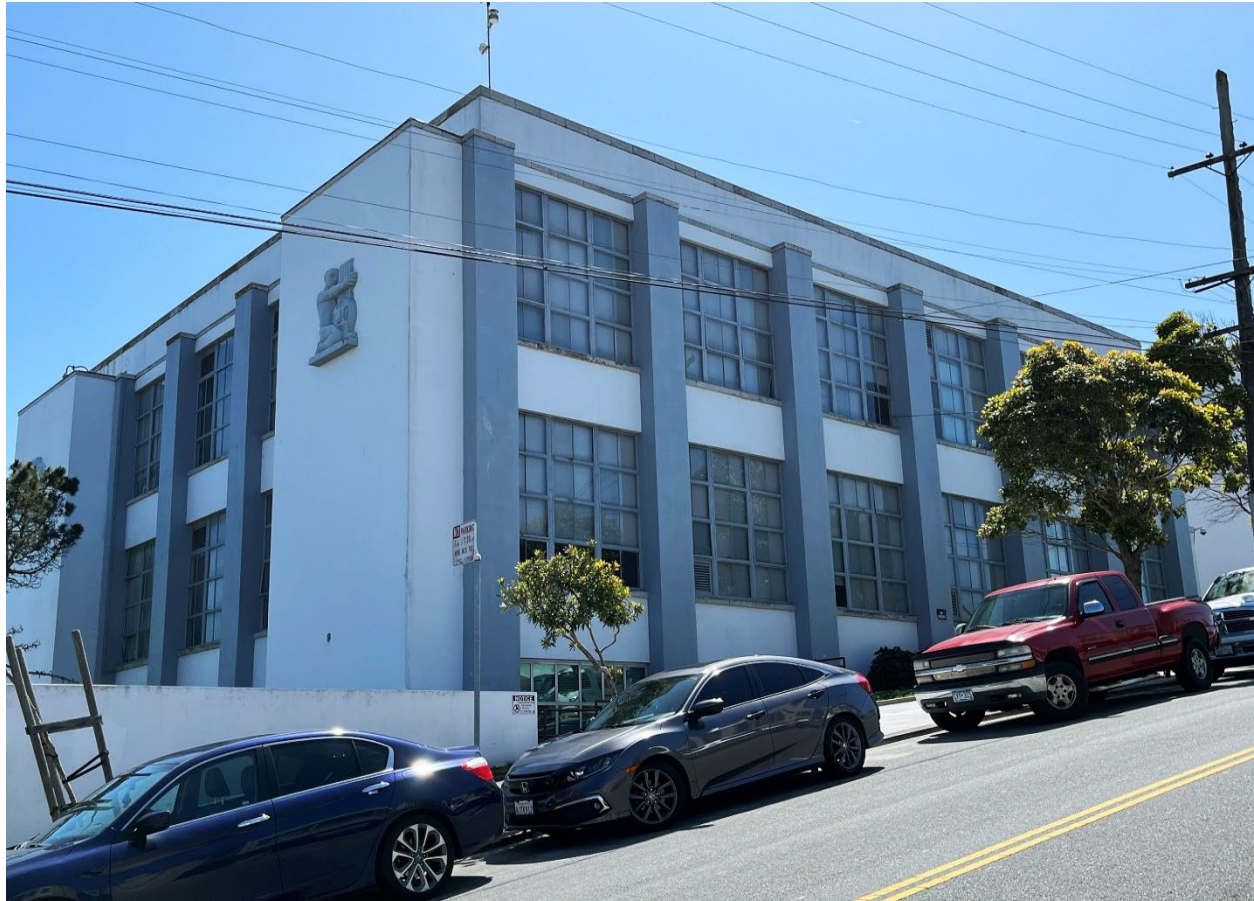
Photo 14. North and west façades of Shop Building, camera facing southeast.
